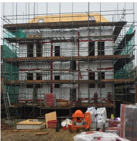
Folkestone – New Build 14 Apartments
